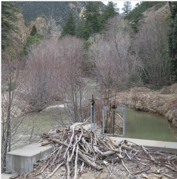
Current South Ditch Diversion structure.
