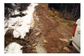
Left: Good water bar (rolling grade dip); Right: No water bar, causing erosion.
