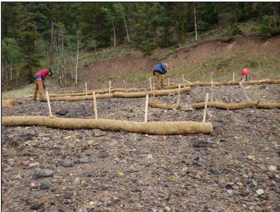
A SCC crew installs straw wattles to control erosion.
