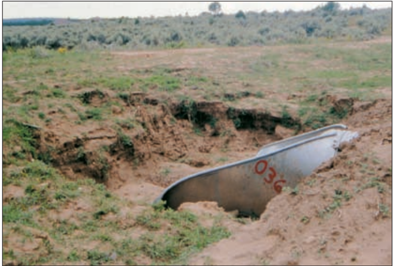
Photo VIII-2: Headcutting caused by improper culvert installation.
