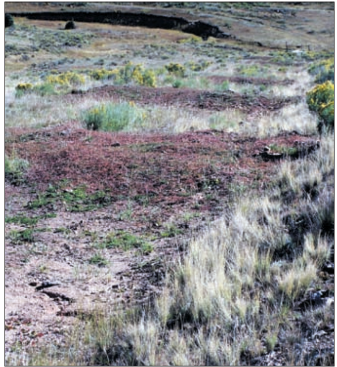
Photo V-5: Water bars are easily flattened and only suitable for abandoned roads or roads closed to traffic when wet.
