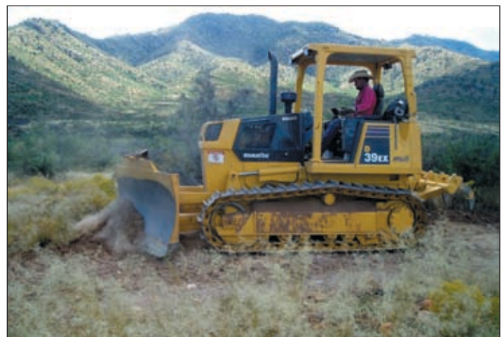
Photo IX-1: A medium sized bulldozer is ideal for building cross drains and for most maintenance situations.
