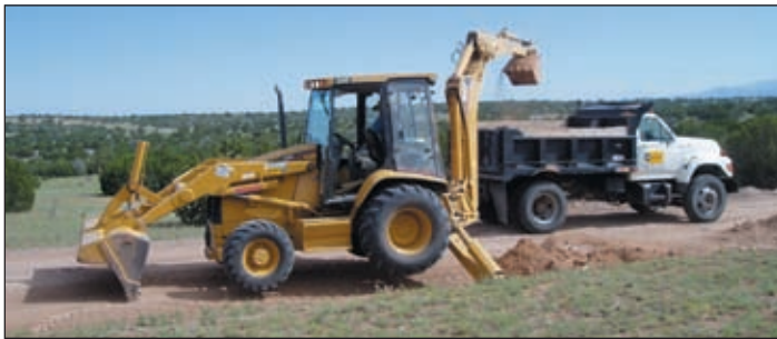
Photo IX-2: Backhoe removing sediment from a culvert inlet.
