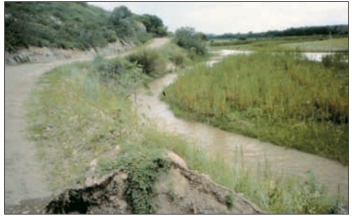
Photo VIII-4: Road encroachment on streambank.
