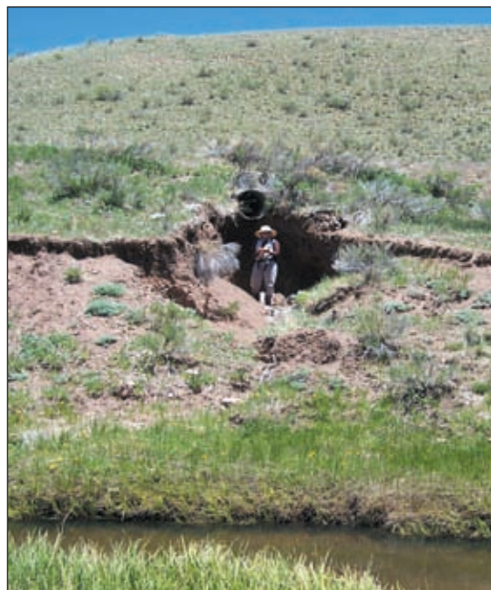
Photo IV-3: This cross drain culvert was installed at a point where the soil could not absorb concentrated runoff and should be relocated to a more favorable site that can filter and absorb road runoff.
