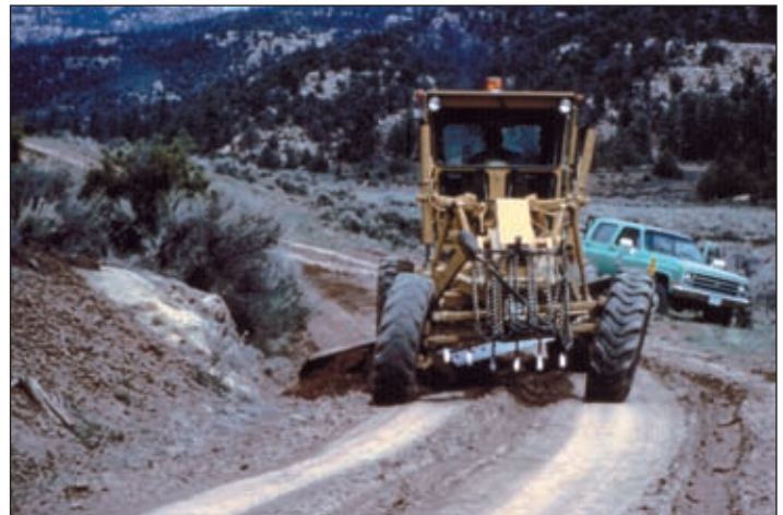
Photo V-3: Blading to maintain an insloped road template.
