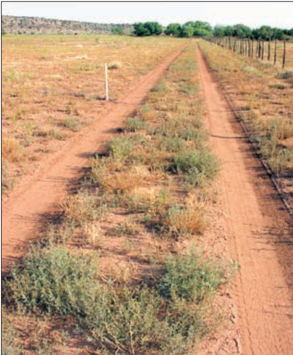
Photo V-8: A flat road on flat land. The stake marks the location of the planned drainage outlet.
