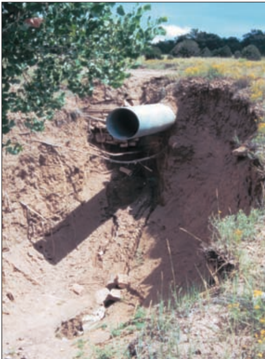
Photo V-12: This 18-inch diameter corrugated steel pipe had adequate cross slope, but no energy dissipater.
