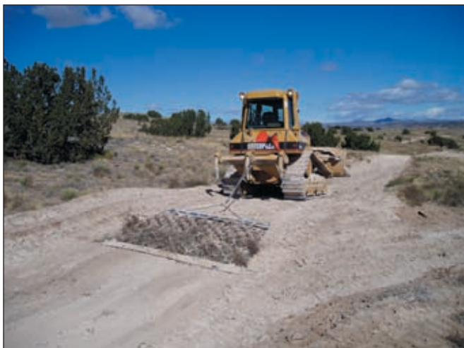
Photo IX-8: Chain harrow pulled behind a bulldozer to smooth a rolling dip.
