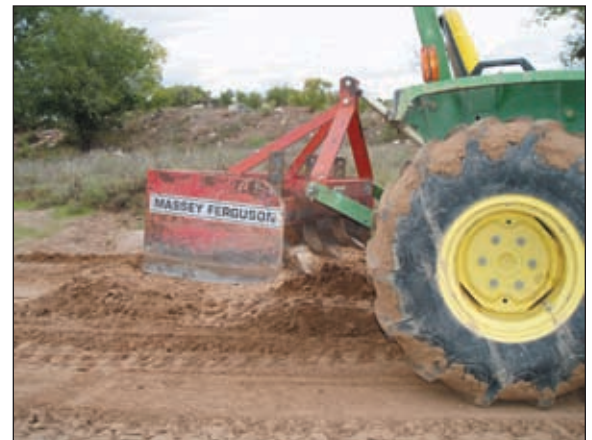
Photo IX-5: Farm tractor with a box scraper and rippers.
