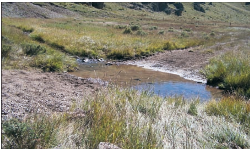
Photo VIII-1: Unimproved fords are commonly used stream crossings on low standard roads. A road should cross at right angles to the direction of the flow to avoid stream capture.
