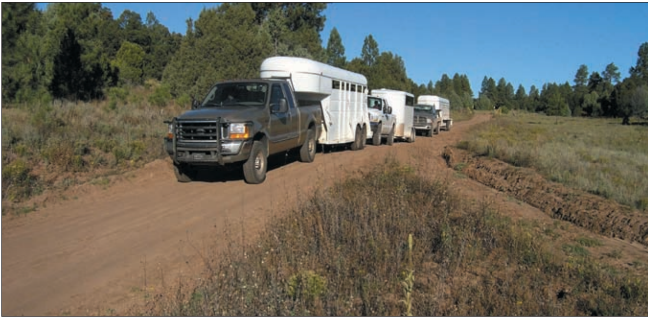
Photo V-6: If the road will be used by a truck pulling a trailer, the dip and roll-out should be long and gentle.
