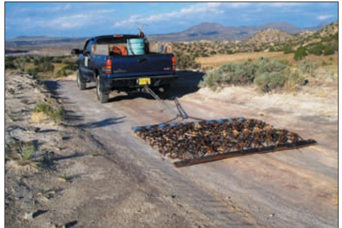
Photo IX-9: Chain harrow pulled behind a pickup to smooth the road surface. Such harrows can also be used to scarify the roadside for seeding.
