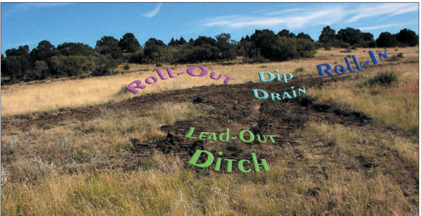
Figure V-3: Key features of a rolling dip are the dip drain, lead-out ditch and roll-out.
