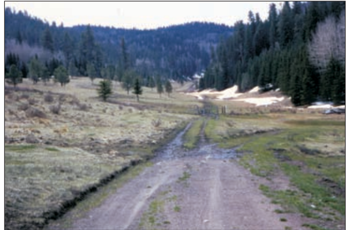
Photo II-1: Valley-bottom roads can be difficult to drain.
