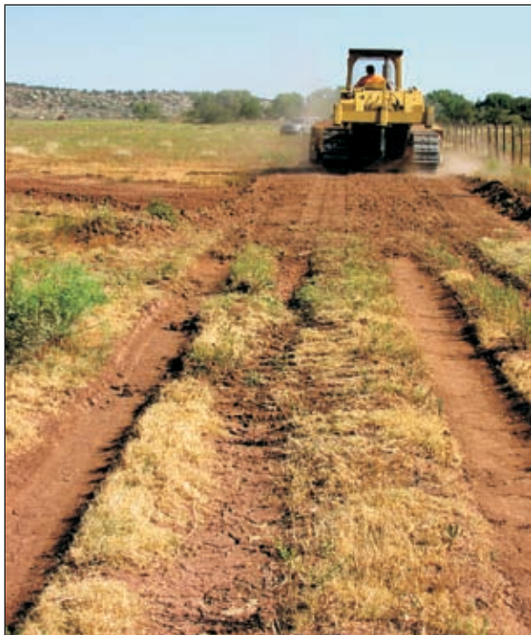
Photo V-10: Tractor constructing reverse slope ramp beyond lead-out ditch using the stockpiled fill (photo V-9).
