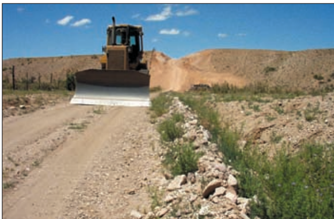
Photo V-1: A crowned road. The berm on the right must be removed to assure drainage to the road ditch.
