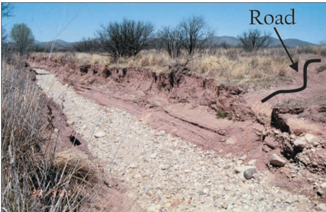
Photo III-2: Straightening of the channel at an unpaved ford caused this channel bed to down cut.
