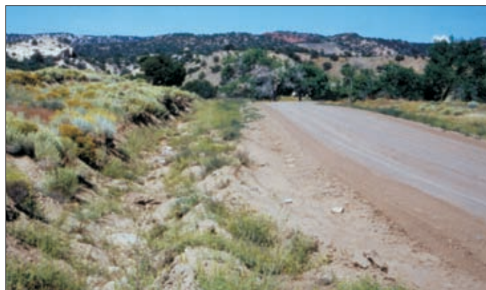
Photo III-1: This berm keeps water from the road surface from spilling into the road ditch.
