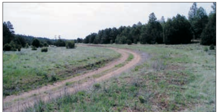
Photo i-2: A low standard ranch road, unsurfaced and without permanent drainage features.
