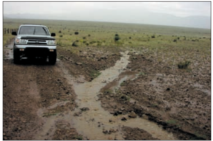
Photo I-4: A rolling dip deflecting water from a ranch road to the adjacent grassland.
