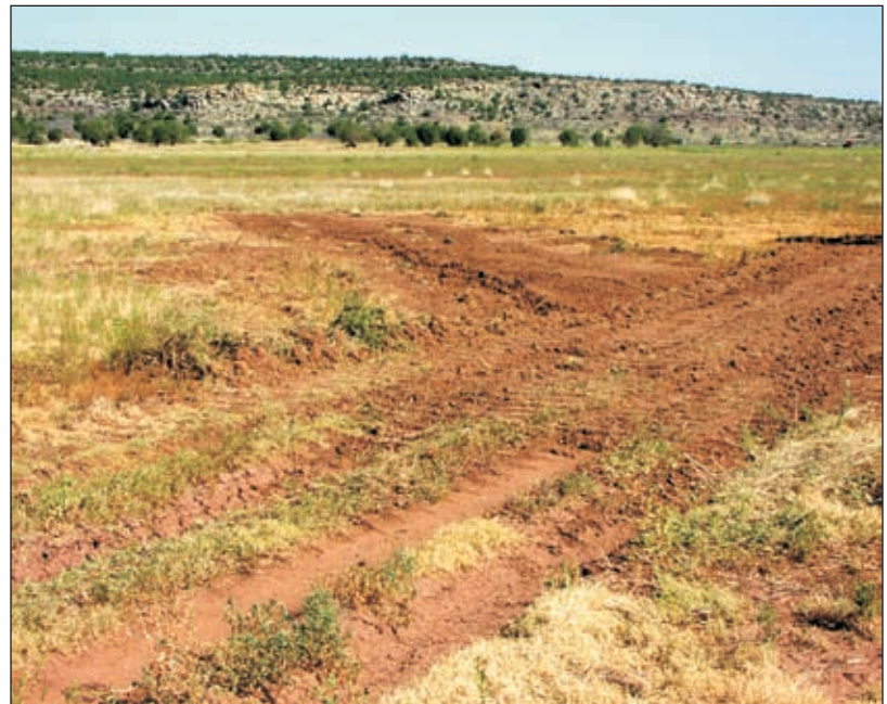
Photo V-11: Completed flat land drain and lead-out ditch on fine-textured soil. If needed, harden the surface with gravel hauled from another source.
