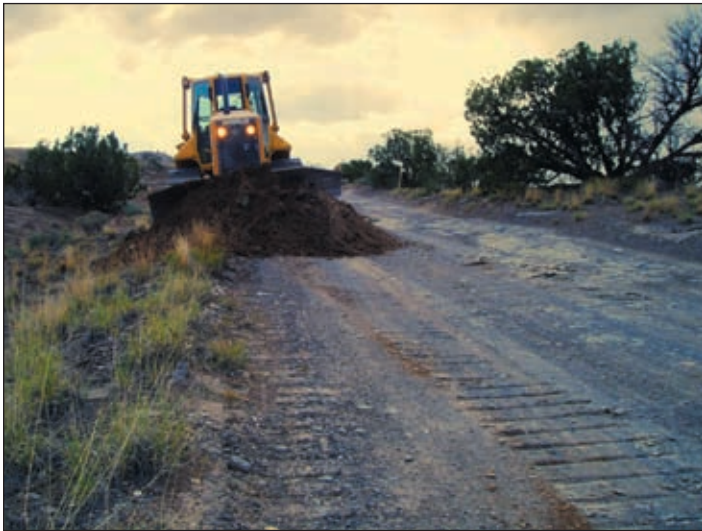
Photo V-4: Removing the unwanted berm will allow surface runoff to spill this outsloped roadway.
