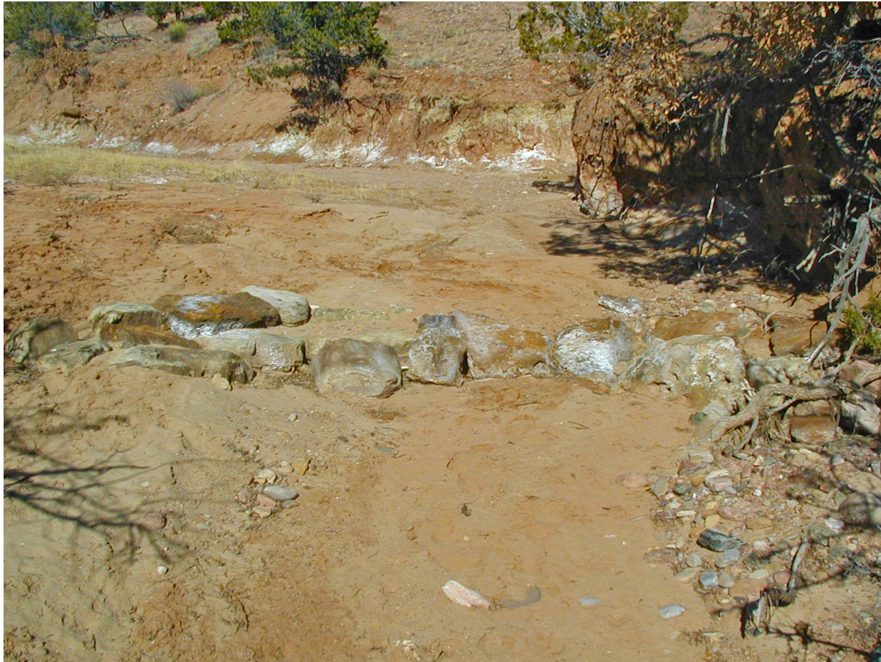
Figure 3.3 Small cross-vane just downstream from the existing wetlands. February 2008. (Photo: Jan-Willem Jansens)
