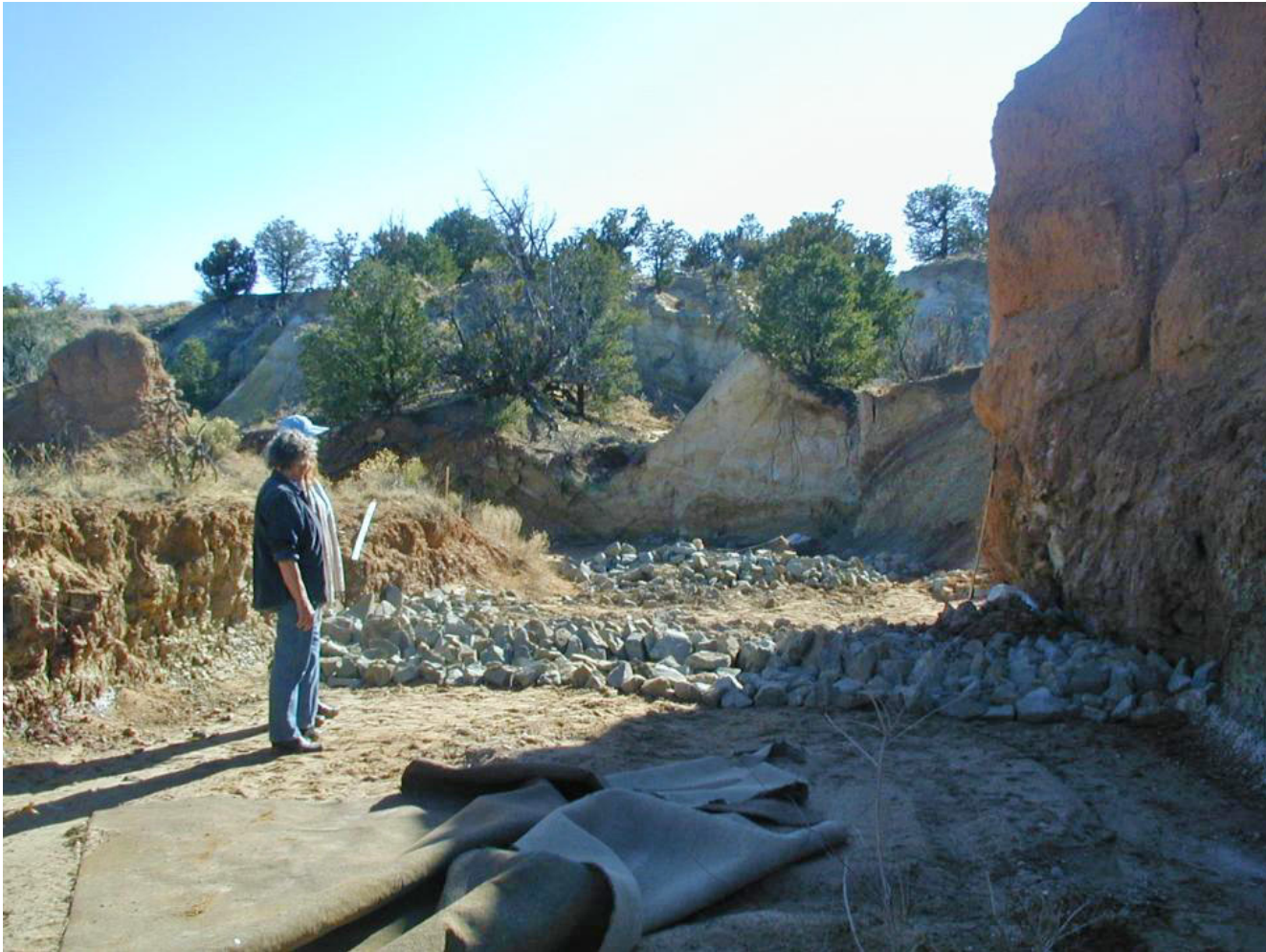
Figure 3.4 Looking upstream across a rock sill. February 2008. (Photo: Jan-Willem Jansens)
