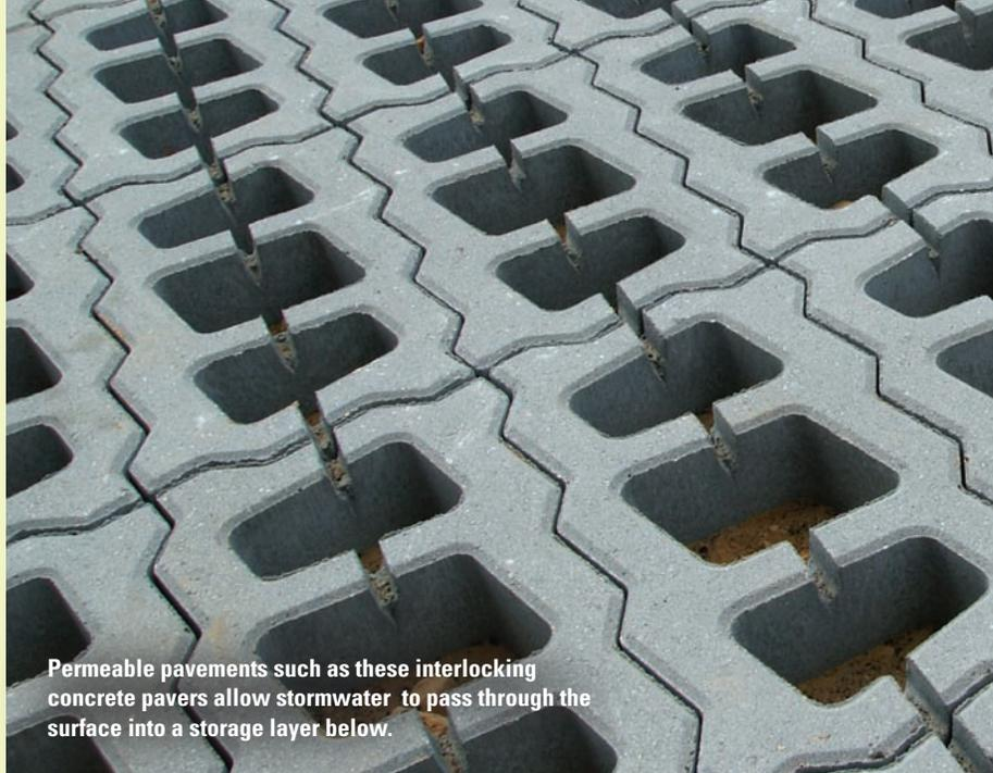
Permeable pavements such as these interlocking concrete pavers allow stormwater to pass through the surface into a storage layer below.
