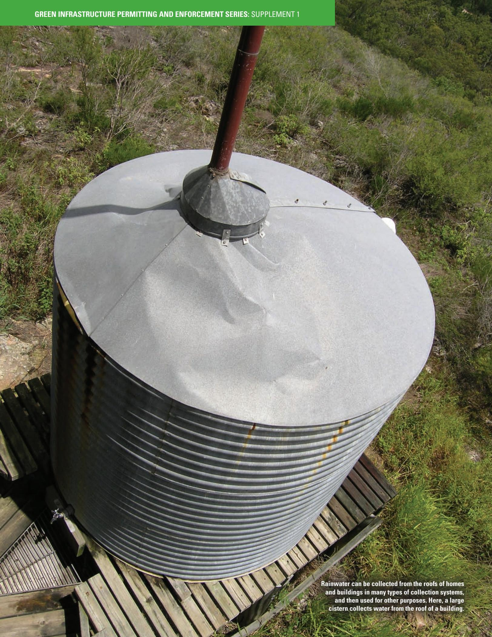
Rainwater can be collected from the roofs of homes and buildings in many types of collection systems, and then used for other purposes. Here, a large cistern collects water from the roof of a building.
