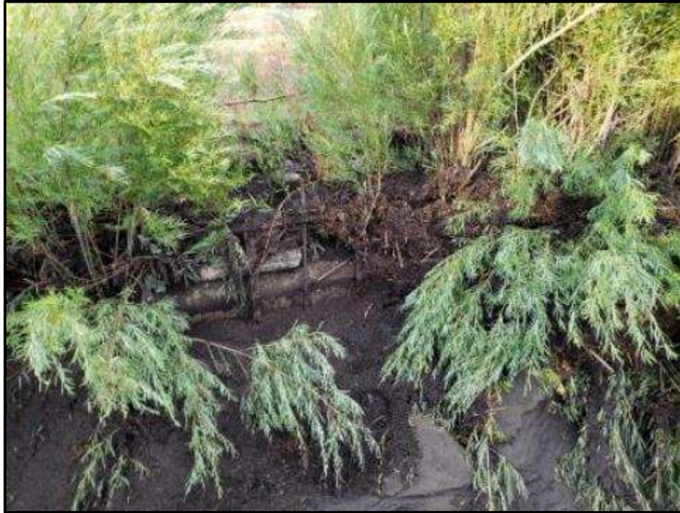
Figure 3.30. View of existing City of Cimarron secondary intake structure.
