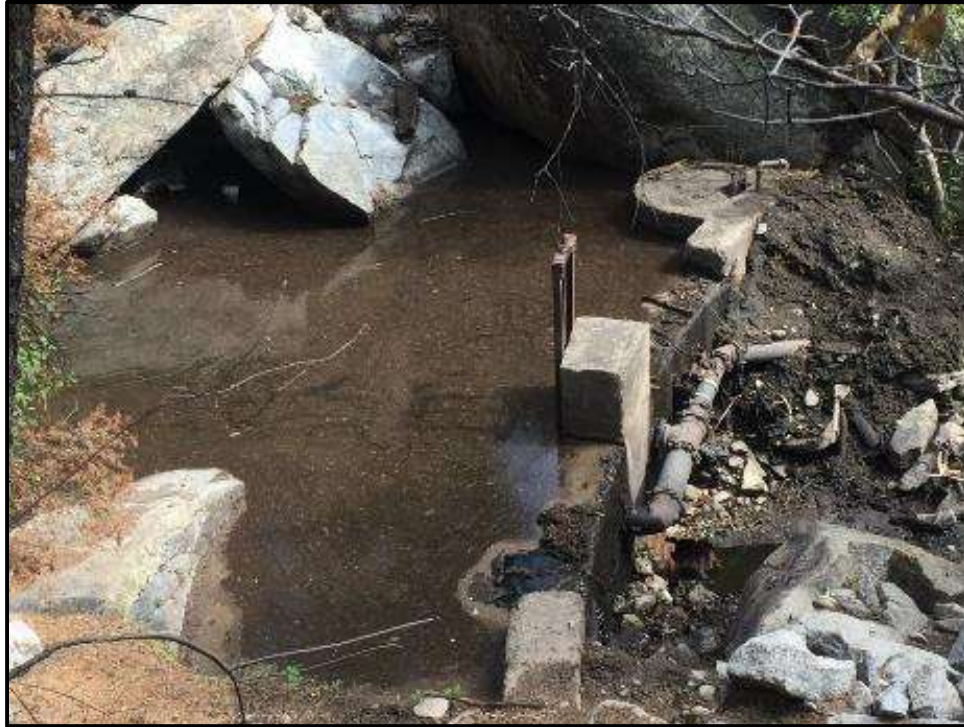
Figure 3.31. View of existing Town of Cimarron intake structure. Notice the pool is black and filled with ash/debris from the adjacent hillslope that received high severity burn.
