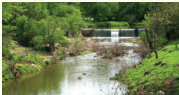
Thousands of low head concrete dams have been built on Texas creeks. These dams disrupt the natural movement of sediment that is needed downstream to build point bars and sinuosity. Erosion is often accelerated below the dams, creating additional problems. Some landowners are now considering the removal of these dams. Photo courtesy of Ricky Linex, NRCS.
