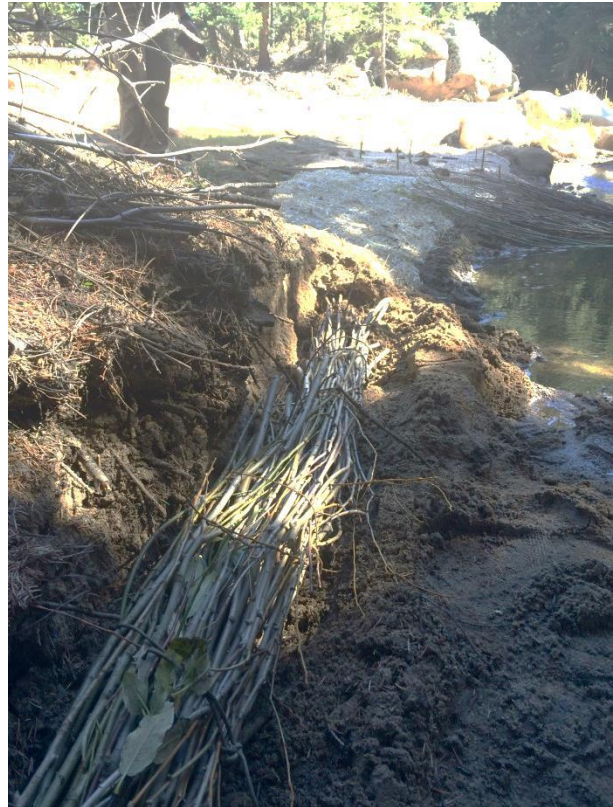
Figure 14. Fascine prior to staking and backfilling, Little Deer Creek, CO. From Giordanengo, J. H. Reprinted with permission.
