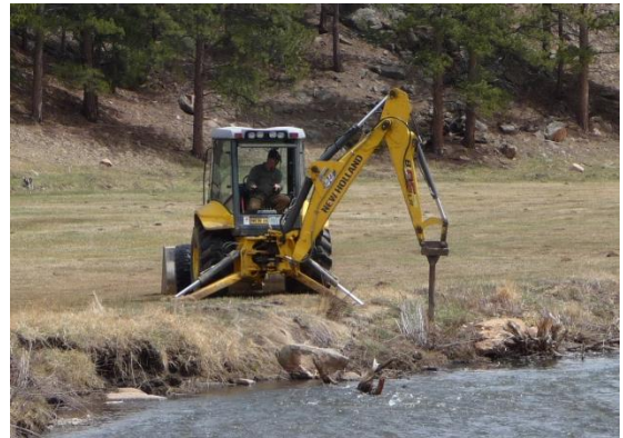
Figure 11. Mechanical stinger probing into the groundwater for willow installation on Tarryall Creek, CO. From Giordanengo, J. H. Reprinted with permission.
