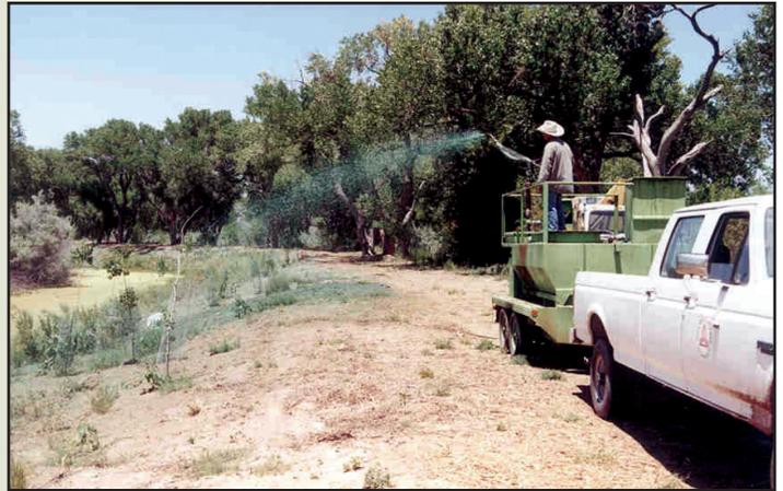
Photo 42 – In July, the site was seeded by hand broadcasting and raking. A wood fiber hydro-mulch was sprayed over the planting after seeding. Plants were temporarily covered during the hydro-mulching activity to prevent them from being coated with the sticky mulch.
