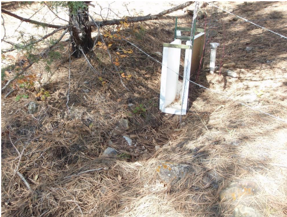
Figure 2.30. Parshall flume located at Chilili site plot 2.
