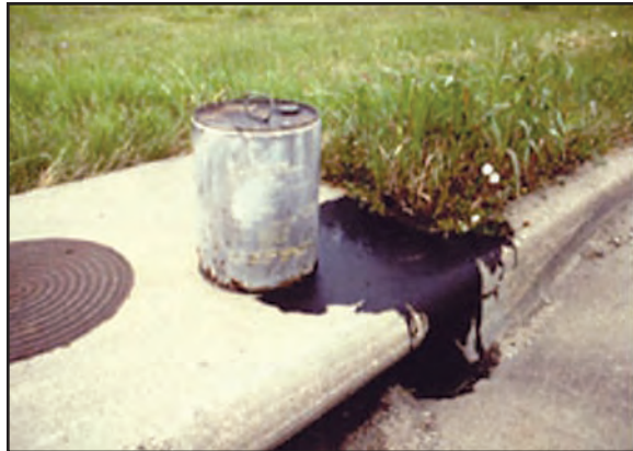
Figure 5: Dumping at a storm drain inlet
