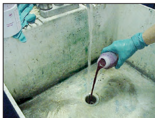
Figure 63: Dye Testing Plumbing (NEIWPCC, 2003)
