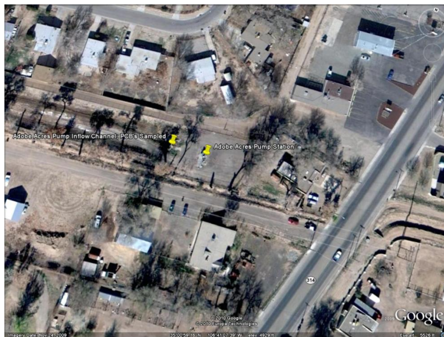
Photo 3. Adobe Acres Pump Station
