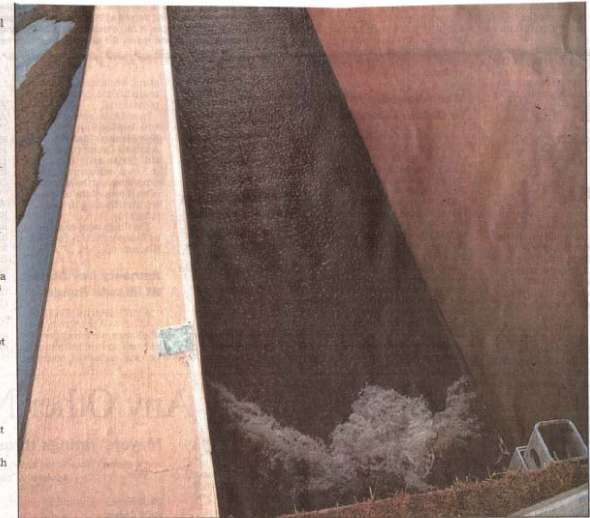
Water from a summer thunderstorm streams into a trap intended to keep empty water bottles and other trash from reaching the Rio Grande.
