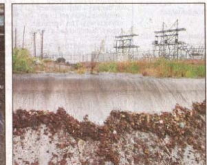
A steel screen in northeast Albuquerque allows stormwater to filter through while diverting floating trash so Albuquerque Metropolitan Arroyo Flood Control Authority workers can keep it from reaching the Rio Grande.
