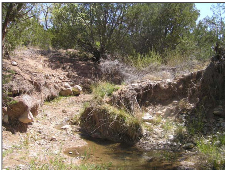
Restoration of deep downcut gully and back-eddy area at Van Driessche/Bladergroen property boundary – (view upstream). Note baffle installation on right and restoration of floodplain. Photos courtesy of R. Bandeen
