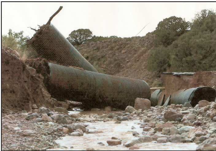
Flood damage on Las Huertas Creek, July 2006
