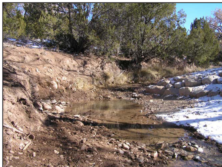
Restoration of deep downcut gully and back-eddy area at Van Driessche/Bladergroen property boundary – (view upstream). Note baffle installation on right and restoration of floodplain. Photos courtesy of R. Bandeen
