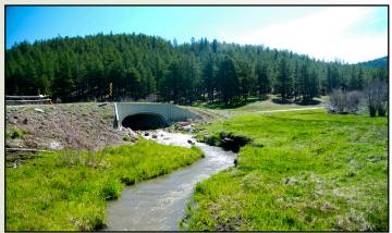
Photo 2 – Rio Guadalupe Bridge Crossing with associated armoring which reduces meandering and increases bank erosion, Sandoval County
