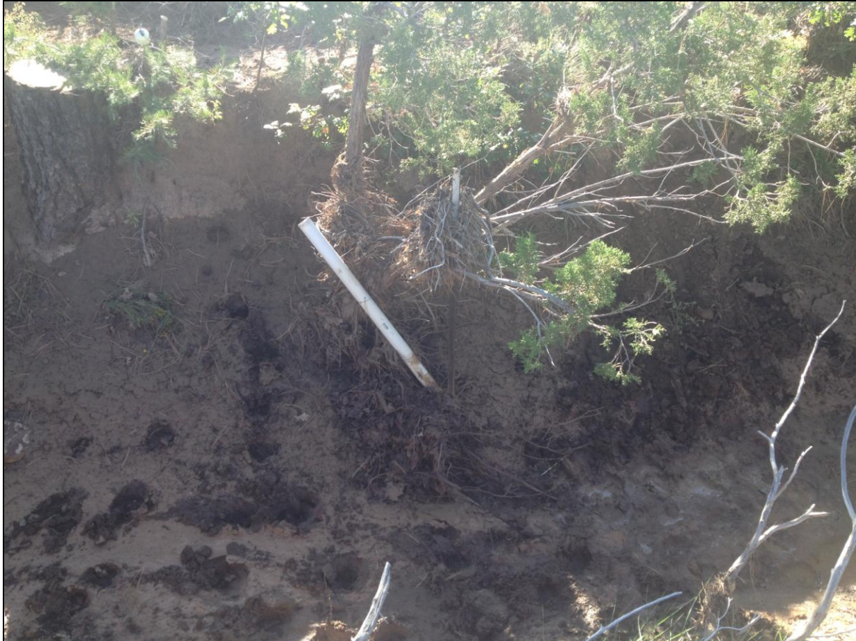
Figure 3.2. The Vigil piezometer in the fall of 2012 after a storm event destroyed the gauge.
