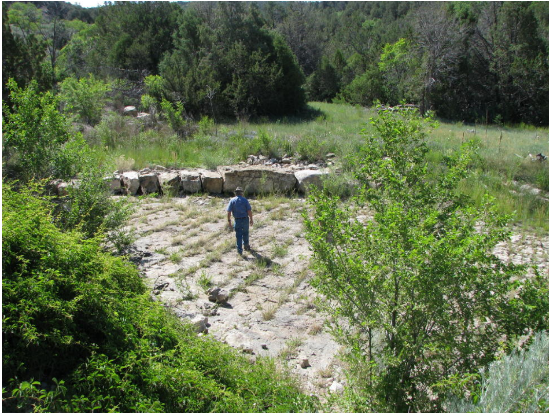
Filter Dam on Cedro Creek
