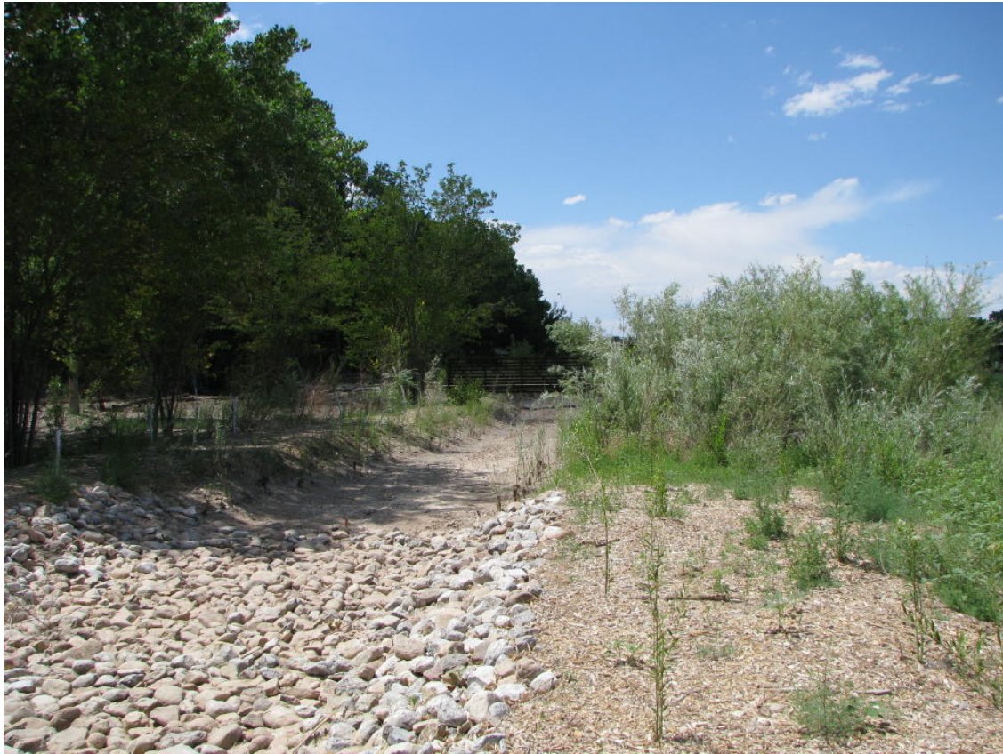
Rock lined overbank canal at Bosque site south of Central Ave.
